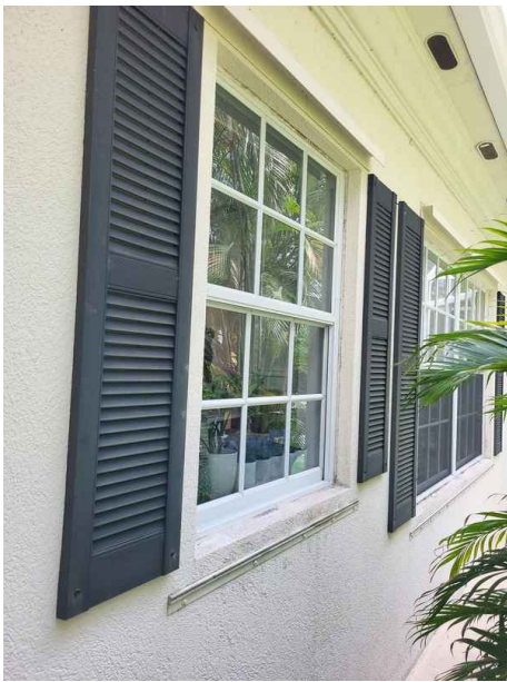
Impact rated shutters (Verified Steel panels)
