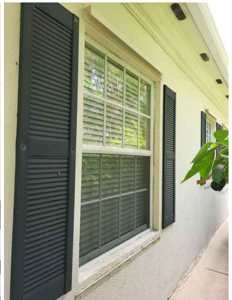
Impact rated shutters (Verified Steel panels)
