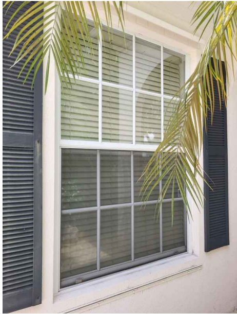
Impact rated shutters (Verified Steel panels)
