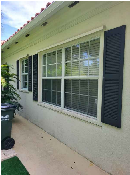
Impact rated shutters (Verified Steel panels)
