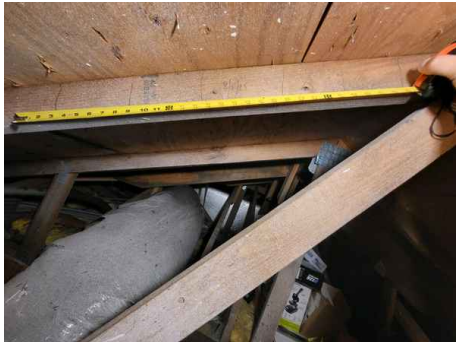
Roof deck attachment with 8d nails spaced max of 6 inches in the field
